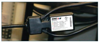
The Z-ATS<sup>m</sup> HV-Y versions allow a single Z-ATS<sup>m</sup> unit to protect 2 or 3 devices from a power failure simultaneously. Please note that the total load of all served devices cannot exceed the rated load of the Z-ATS<sup>m</sup>.
